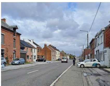
Figure 67; Chaussée de Thuin, 291. Source : Agora
